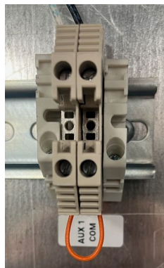
Figure 7 – Aux 1 Input Terminals
